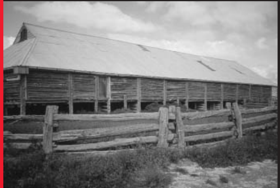
This pine log woolshed at Mungo Station in the western districts of New South Wales is believed to have been built by Chinese rural labourers in 1869. (D Robin, AHC Collection)
