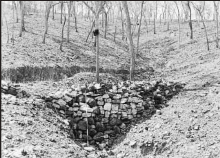
This stone retaining wall was constructed by Chinese alluvial gold miners on a gully off Butcher's Creek in Queensland's Palmer goldfield. Its purpose was to divert upsteam water into two races heading in differing directions. (J Wegner)
